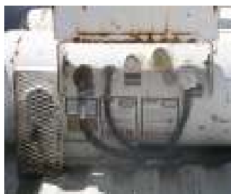
Fuel line Connections
