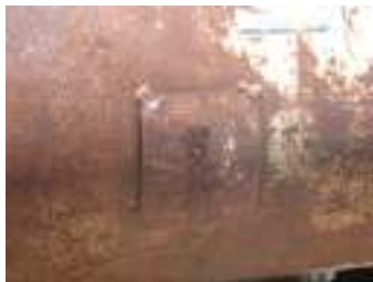
Corroded & Unreadable fuel tank data plate
